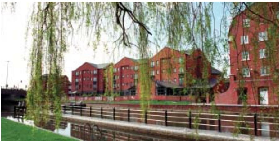
Holybrook Development, Reading
